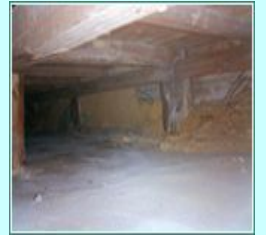
= 床下点検 = 湿気でカビだらけ
